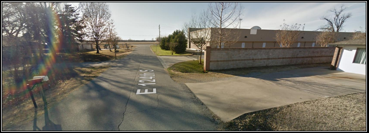
Figure 7: VIEW OF BACK SIDE OF PUD 29A FROM E 124 TH STREET
