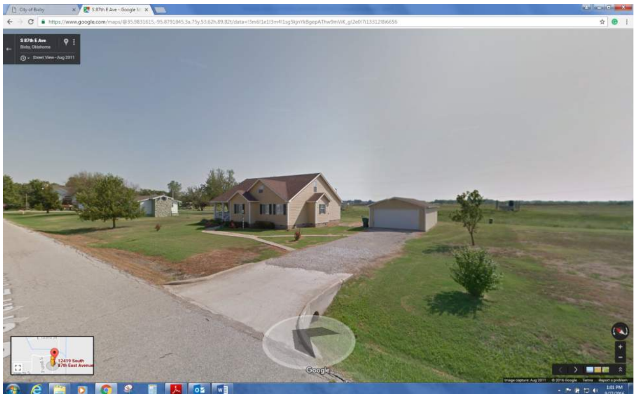
Figure 7-GOOGLE: SUBJECT PROPERTY LOOKING NORTHEAST (BEFORE INITIAL CONSTRUCTION OF FENCE)
