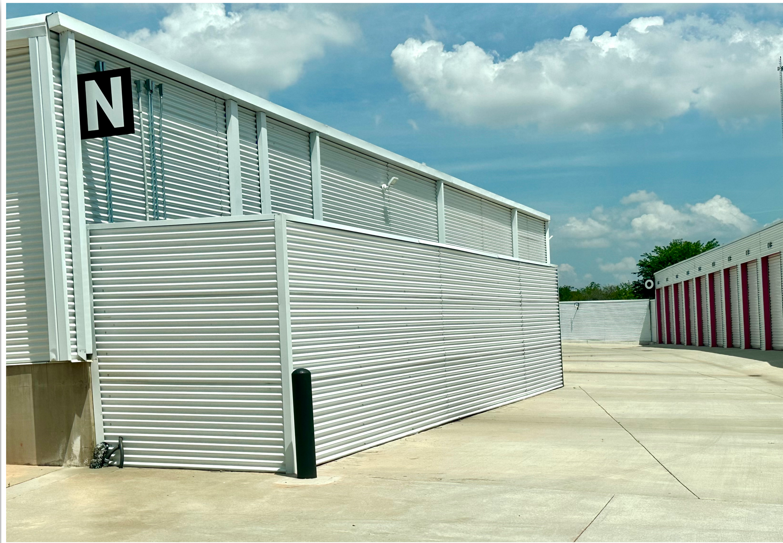
Dumpster Enclosure Blind
