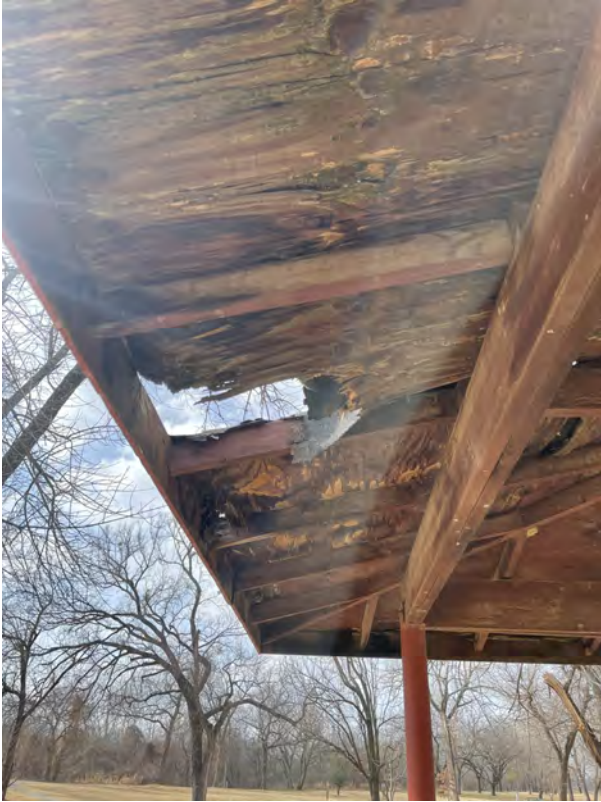
Damaged decking
