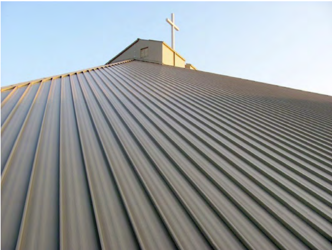
Standing seam metal roofing system
